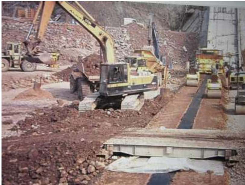
Figure 10. Simultaneous compaction of asphaltic core and filters ( Høeg, 1993 )
