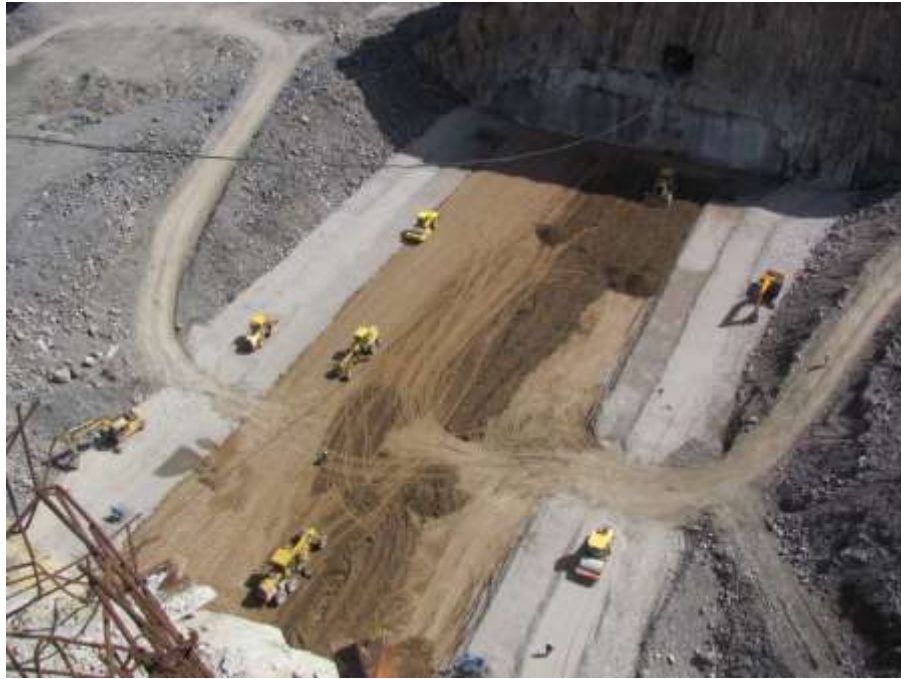
Figure 15. Rudbar-Lorestan Dam under construction.( courtesy Martin Wieland )
