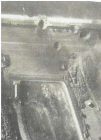
Figure 9. Sorpe dam after heavy bombing in WWII.
