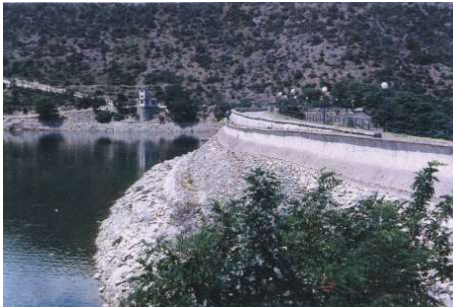
Figure 3. Tikves dumped rockfill dam in North Macedonia.
